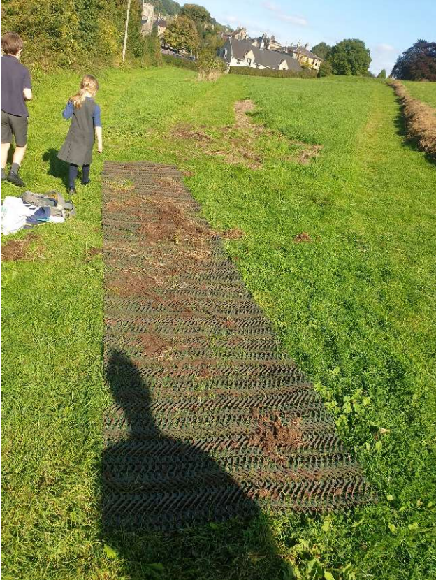
Test section of matting removed by the Tynning gate
